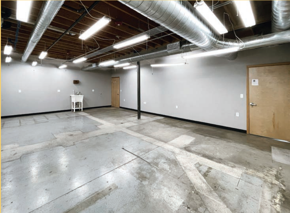
FIRST FLOOR LAB SPACE
